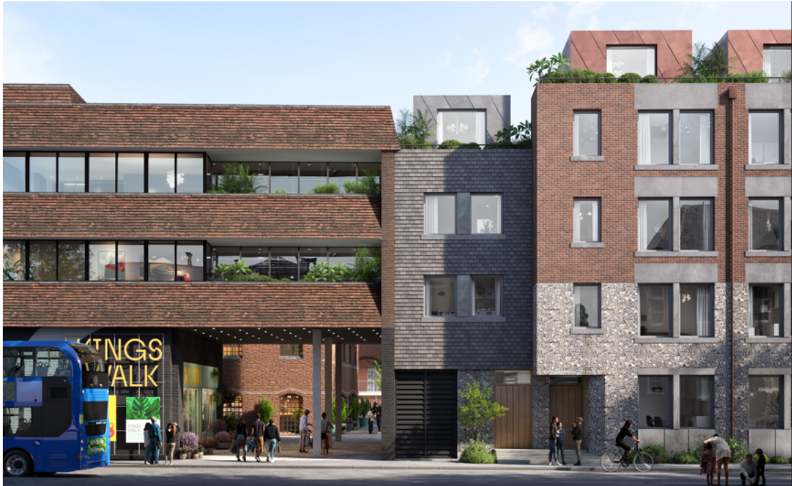
Looking west from Tanner Street through to the Antiques Market and the Brooks Centre
